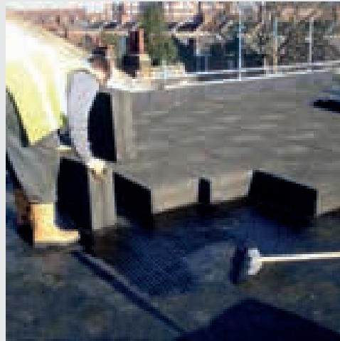
FOAMGLAS® flat and tapered insulation can be used on concrete, timber and metal structures
