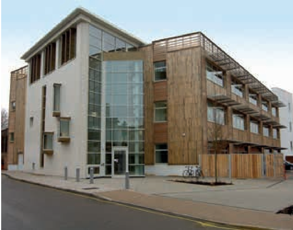
Façade, timber cladding
