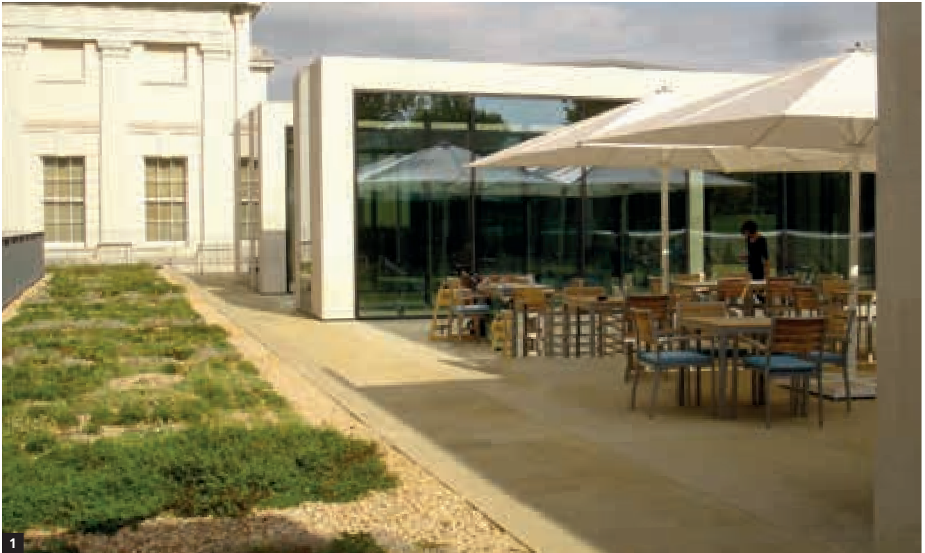
1 National Maritime Museum, London, Gallery roof and restaurant terrace. Architects: Purcell Miller Tritton.
