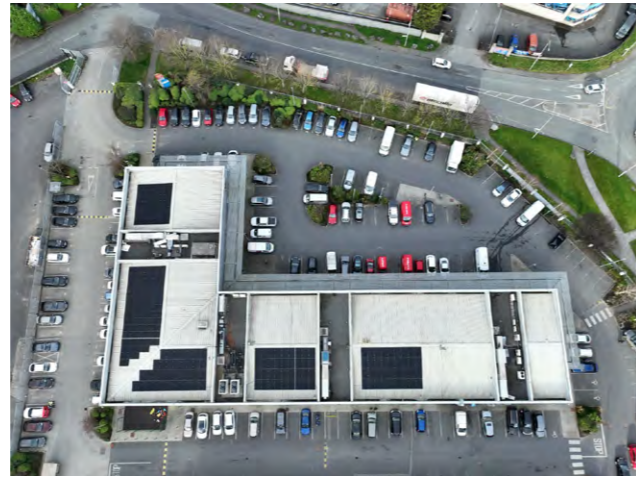
Drone photo of solar panels on our Head Office in Ballymount
